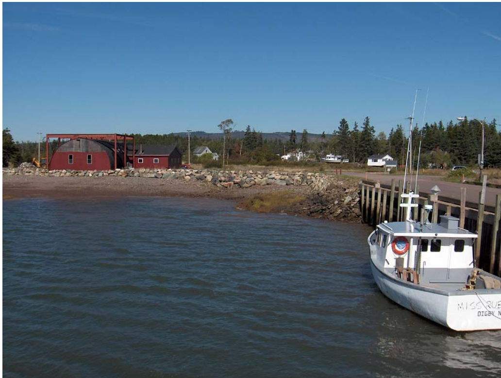
Figure 5.1-10 Potential work building just north of Parrsboro public wharf.
