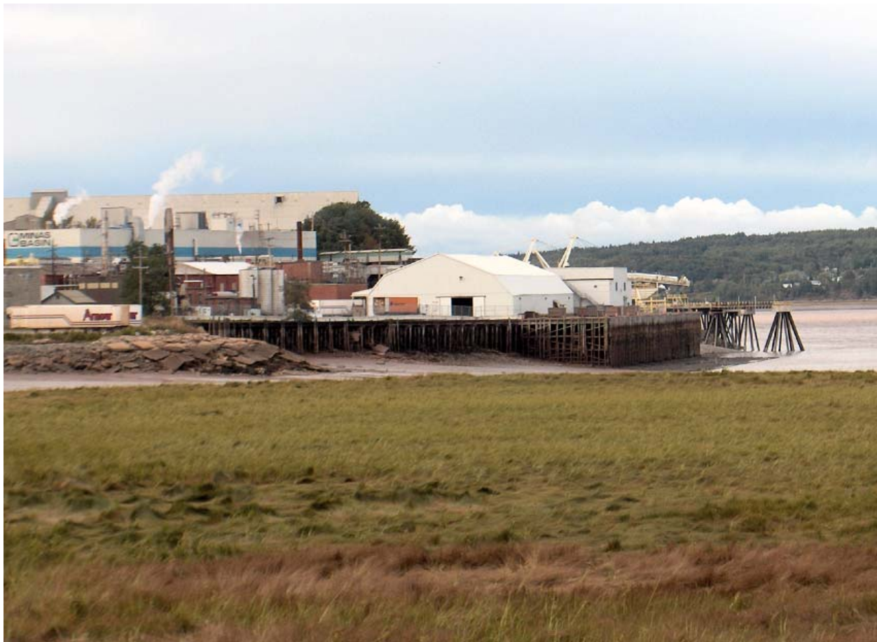
Figure 5.1-11 Hantsport waterfront facilities, looking north. Fundy Gypsum Company pier is visible at right, behind public wharf. Note vessel bed alongside public wharf at water's edge. Minas Basin Pulp and Power Company buildings dominate left side of picture.
