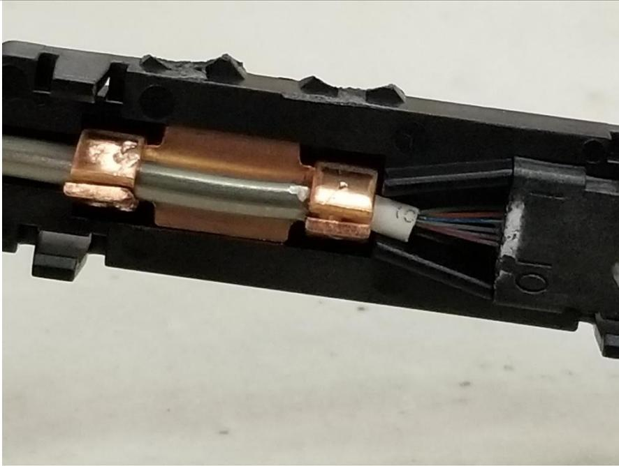
6. Break out kit sealed. Rigid acrylic tubing slid over break out and copper conductors. Fibres fed individually through loose yellow tubing. Silicone application to follow on end of acrylic tubing end.
